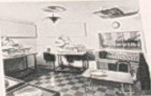
Control room, one RCA Victor Chicago recording studio.
