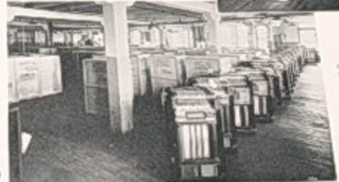
Final Inspection Under the sharp eyes of a trained inspector, a Symphonola is put through a final examination. Lighting, cabinet construction, tuning performance and amplifying system must prove flawless before it is pronounced "O. K."
